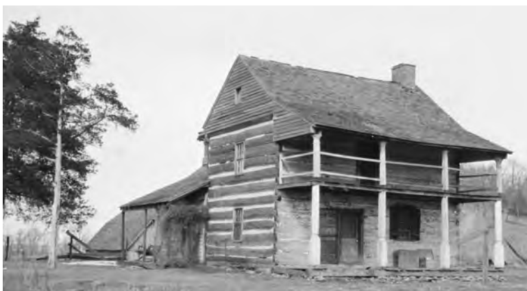
William Logan built this cabin in Fairfield Township before about 1810. Threatened by the construction of the Brookville reservoir in the 1960s, the cabin was moved to Dunlapville. (Photographed ca. 1934, Historic American Buildings Survey, Library of Congress Prints and Photographs Division)
